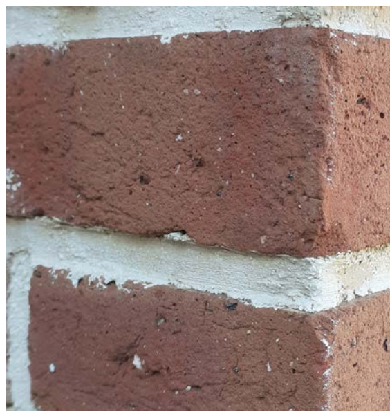
Efflorescences
